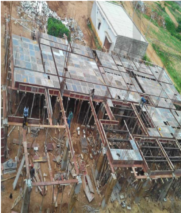
Semi conventional formwork
