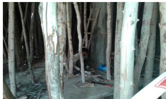
Wooden formwork
