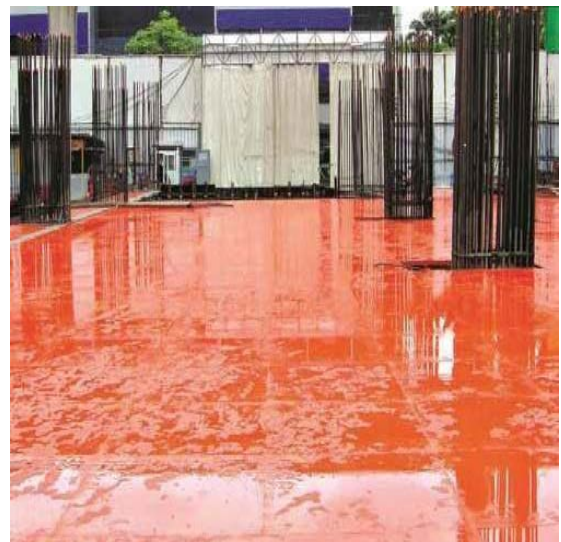
Plastic formwork floor completion
